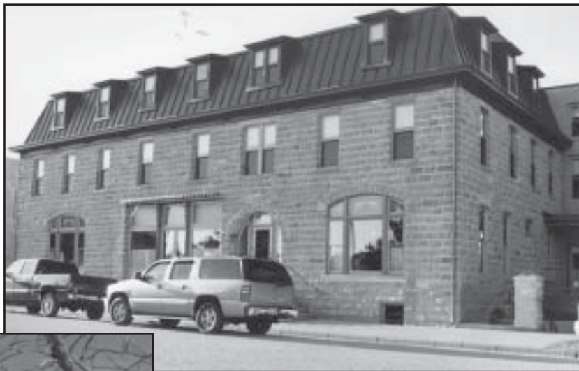
(Right) The Midland Hotel in Wilson was rehabilitated and reopened as a hotel in 2003.
