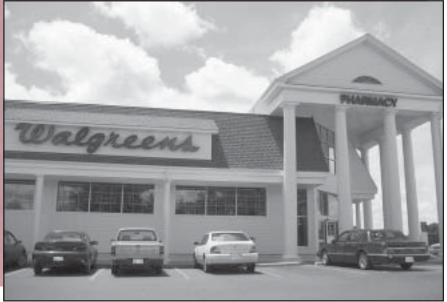
This Walgreens store replaced the Fleming Mansion at the southwest corner of 10 th and Gage in Topeka.
