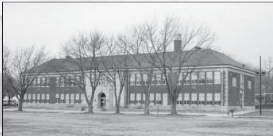
View of the Monroe School following its restoration. Photo courtesy of National Park Service.
